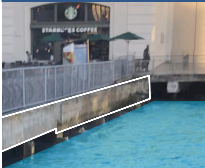
WHARF TODAY AT CURRENT WATER LEVEL
