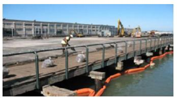
Floating boom is deployed around construction work to capture debris.
