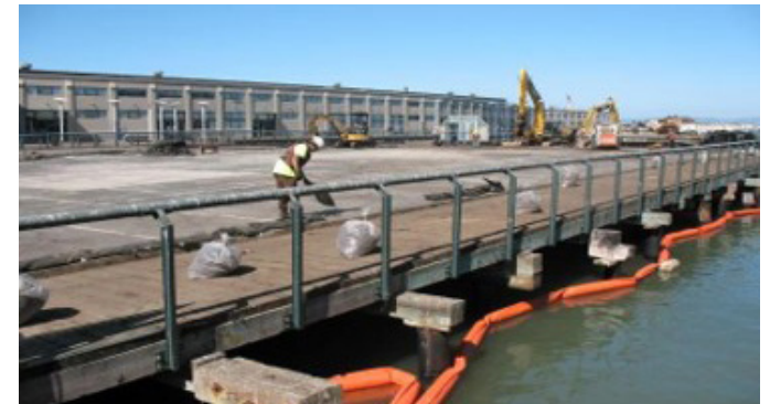
Floating boom is deployed around construction work to capture debris.
