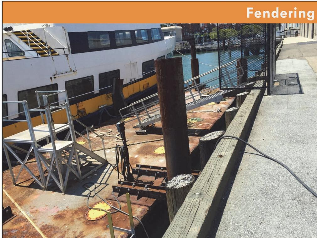
Lay-berth not ADA compliant for passengers. This is a working-berth. Note that windows would be damaged on fender pile – specialized fendering attached to barge is necessary.
