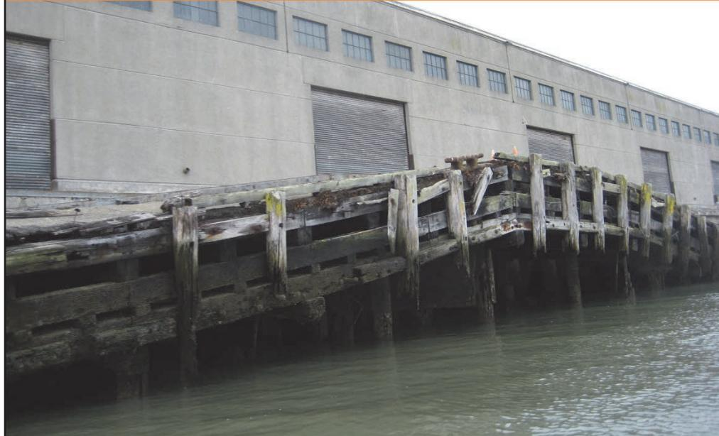
Piers alone are insufficient for berthing: The pier “aprongs” must be in good, sturdy condition.
