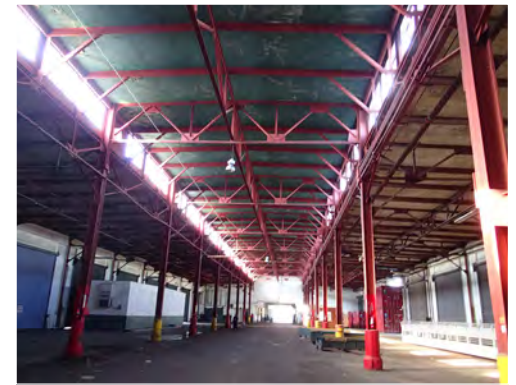
TOP The roof is Spanish-tiled with wood bargeboard and carved purlins and rafter ends. Pier 38 is the last remaining bulkhead in this style. BOTTOM The shed has a steel frame and steel steel trusses and I-beams support the concrete roof.
