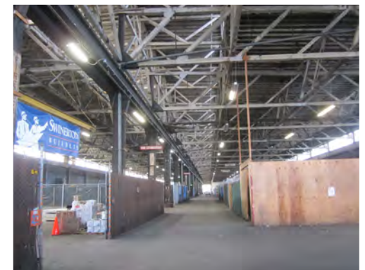
TOP With a water depth of 12-15 ft. vessel berthing may occur alongside, as with most facilities in the RFI. Pier 26 is located just east of energized Transbay and Rincon Hill Neighborhoods. BOTTOM The transit shed is structurally mixed with steel columns and heavy timber trusses.
