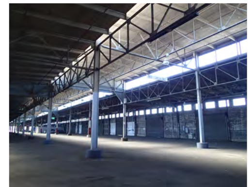
TOP If combined, Piers 19, 19½, & 23 would have 308,000 sq. ft. of floor area. BOTTOM Piers 19 & 23 have wood roofs resting on longitudinal and transverse steel trusses supported by I-beams.
