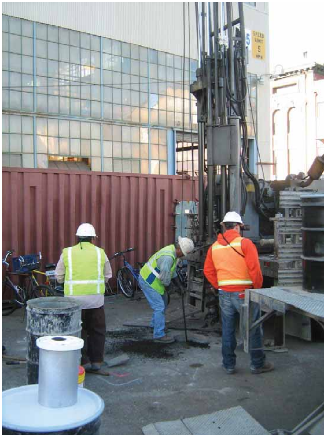
Photograph 2 – Utility Clearance BAE, Parcel 9
