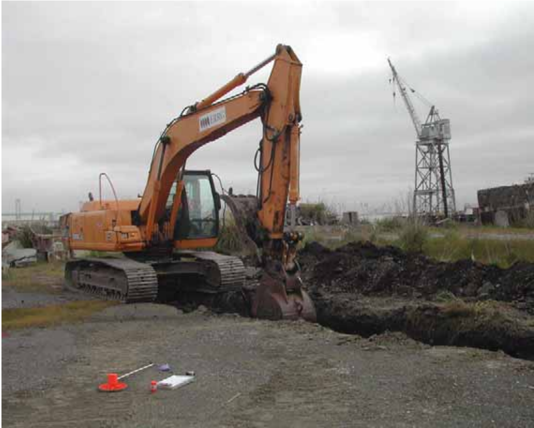
Photograph 7 - Crane Cove Test Pit Sampling, CCTP-01
