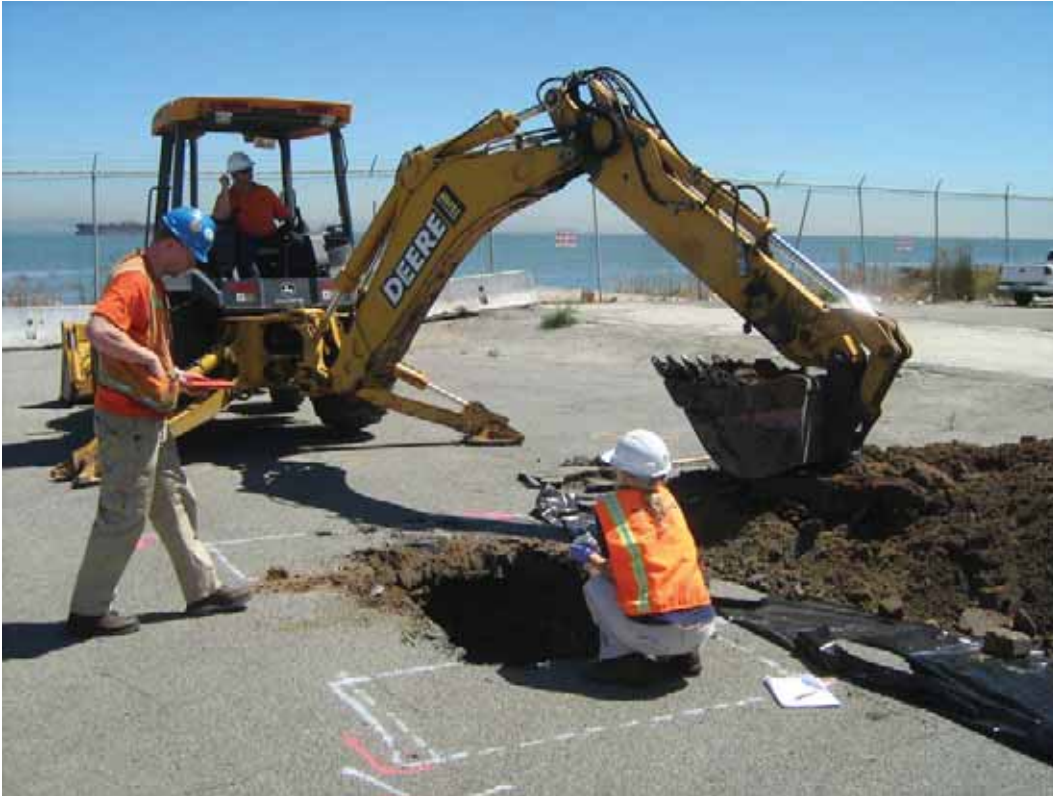
Photo 5 - Test Pit Sampling Slipway Park
