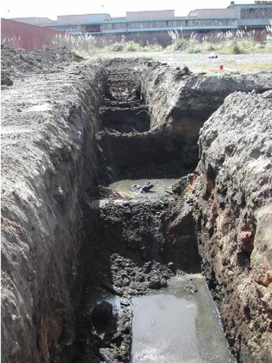
Photograph 8 - Trench of former slipway, CCTP-01
