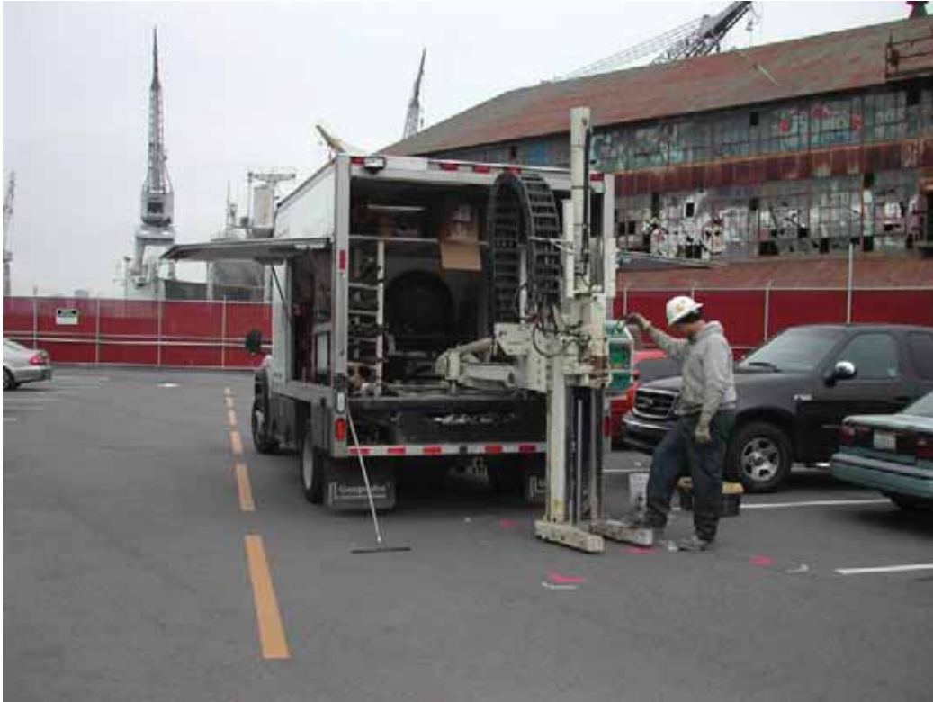
Photo 1 - Direct Push Drilling at the BAE, Parcel 9
