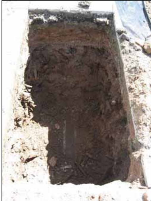
Photo 3: SPTP-03, excavated test pit, concrete slip visible in base of trench.
