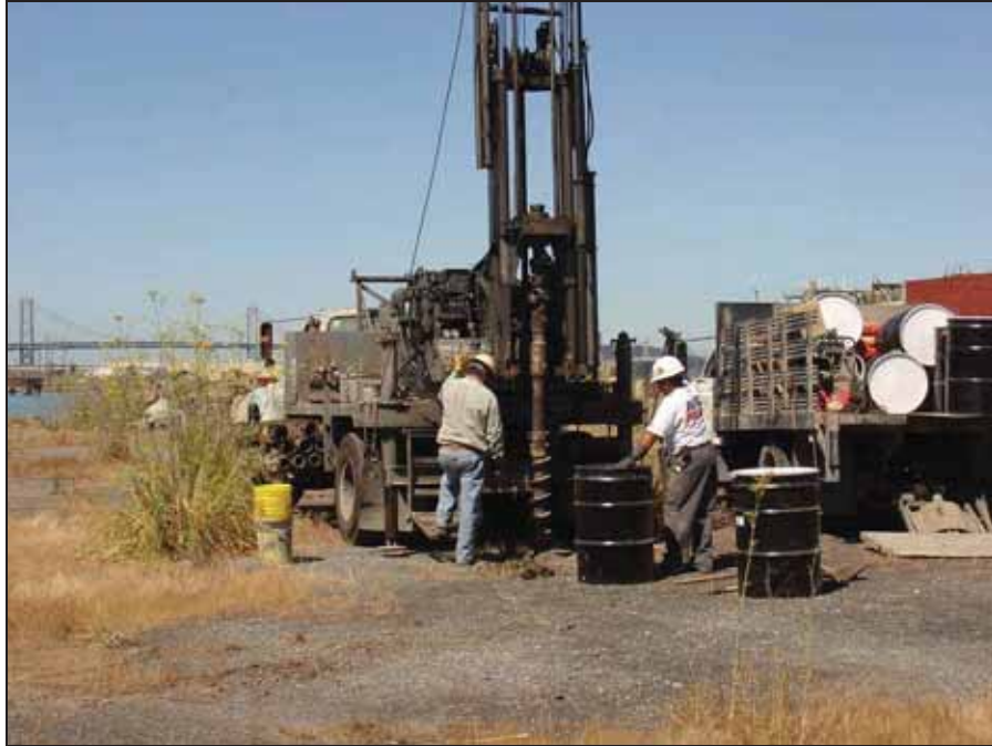
Photo 1: Drilling of CCSB-03 within Slip No. 3, view north.
