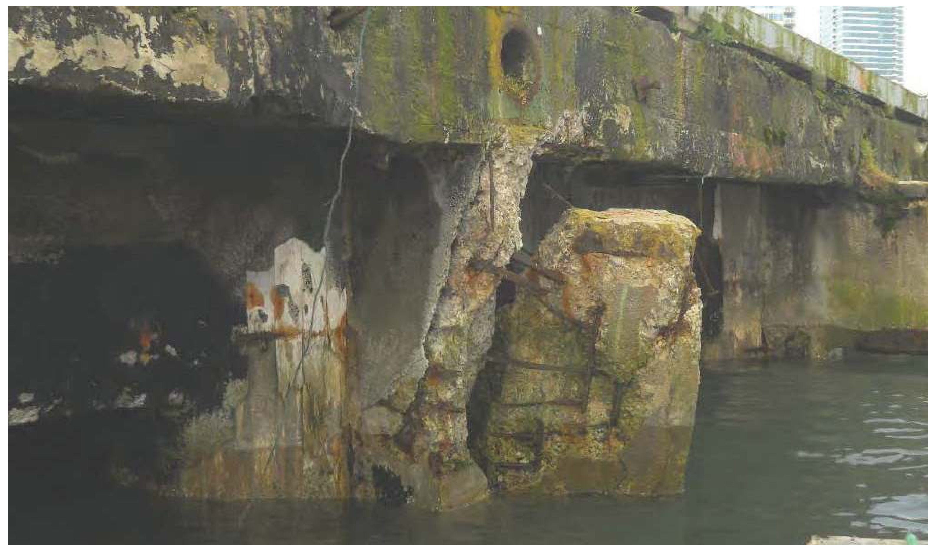
Failing piles
