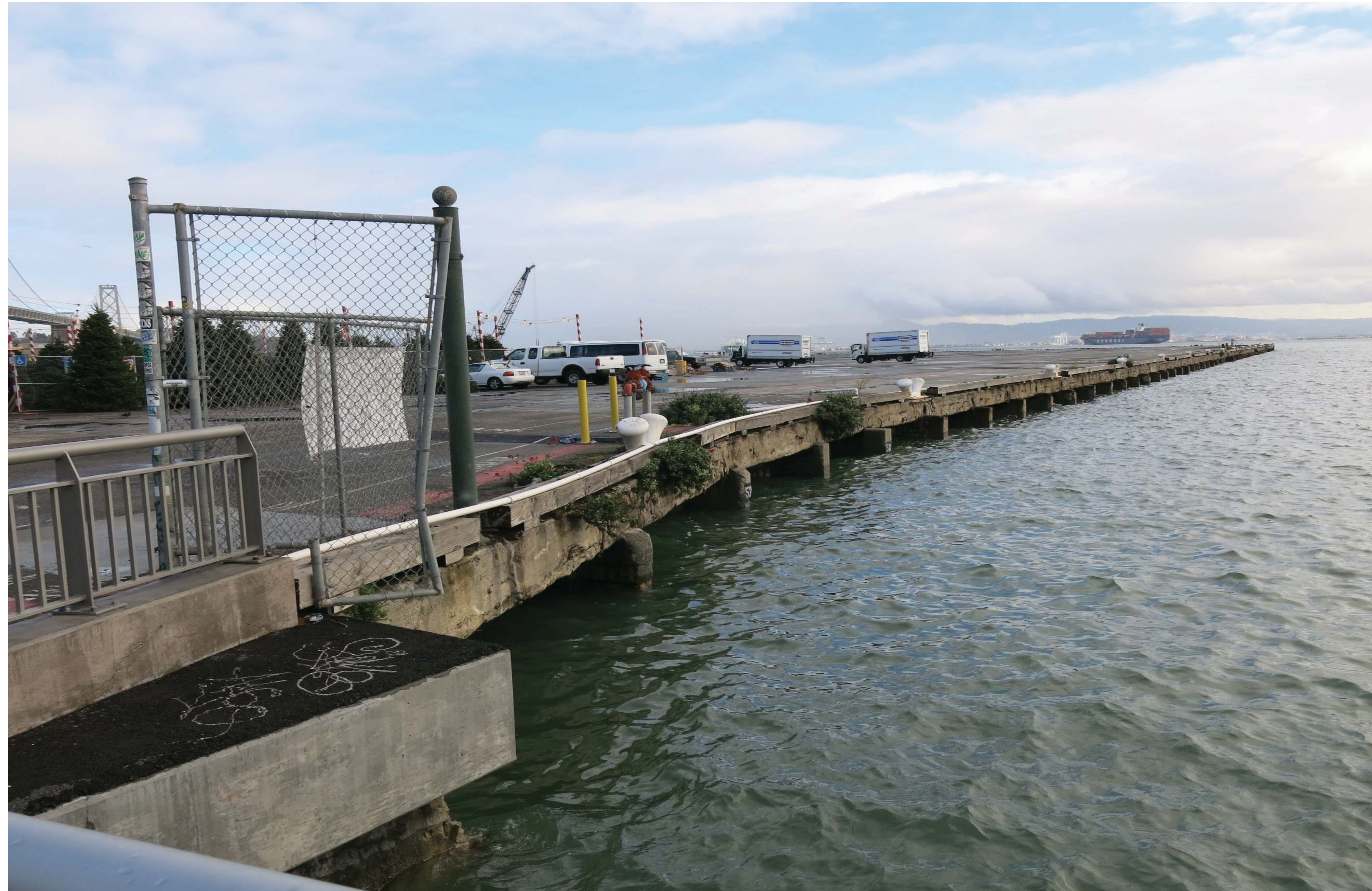
The structural integrity of the Piers varies by location
