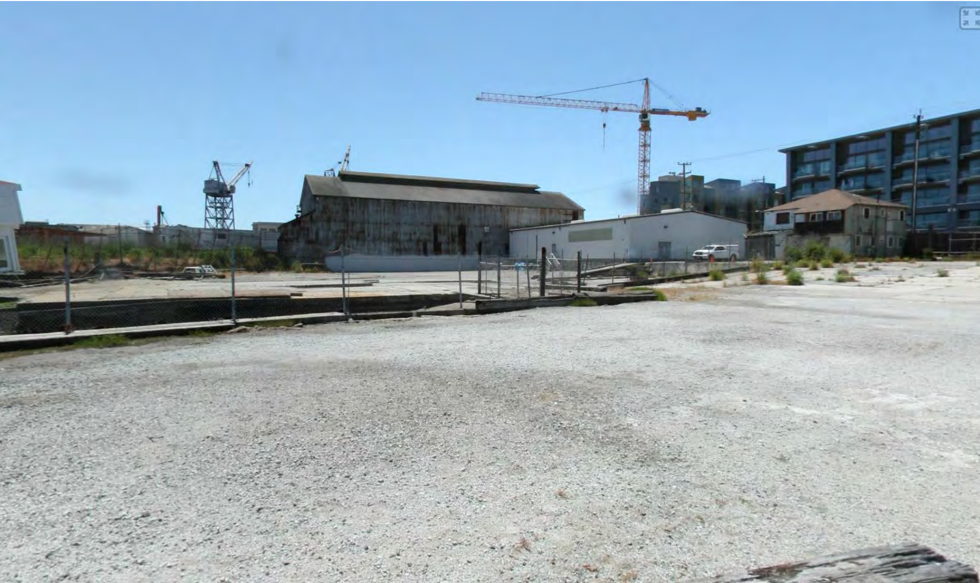
view of un-engineered fill looking south
