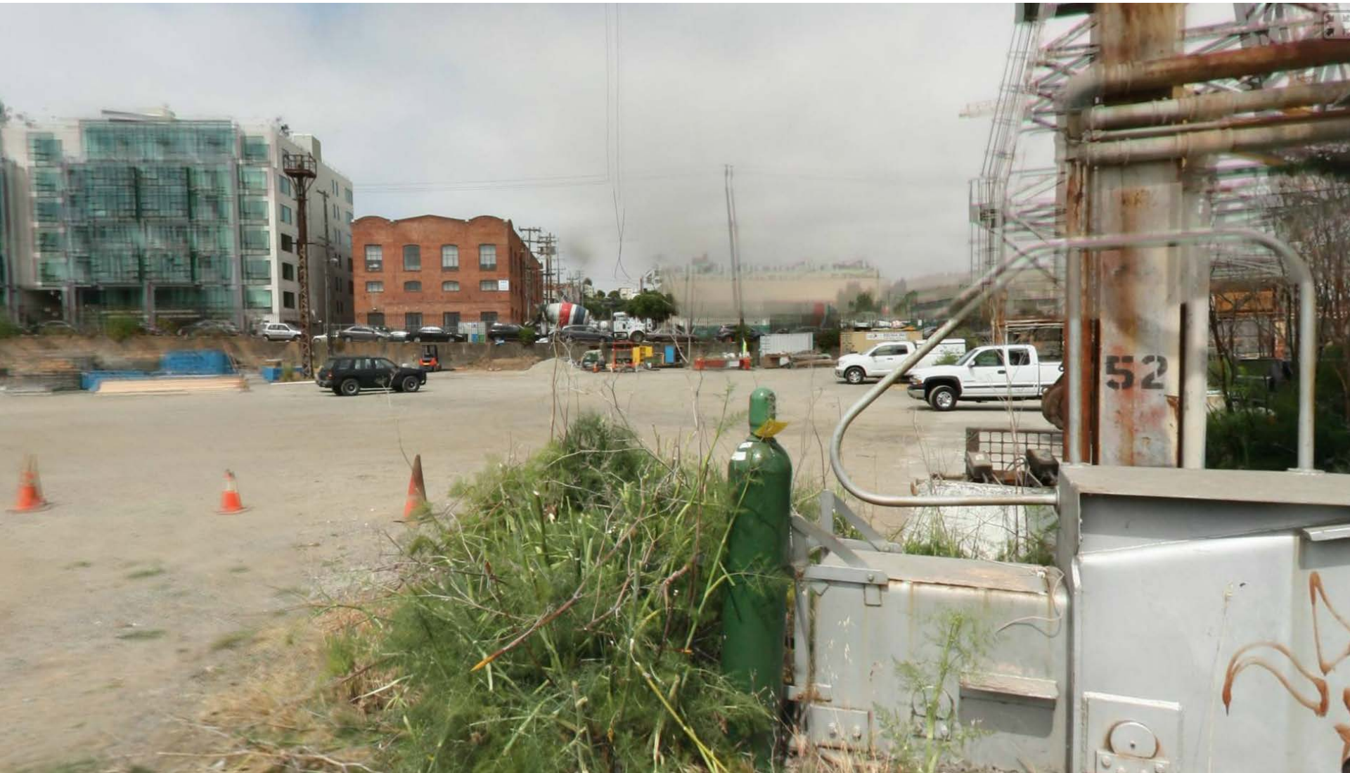
view at eastern runway facing west
