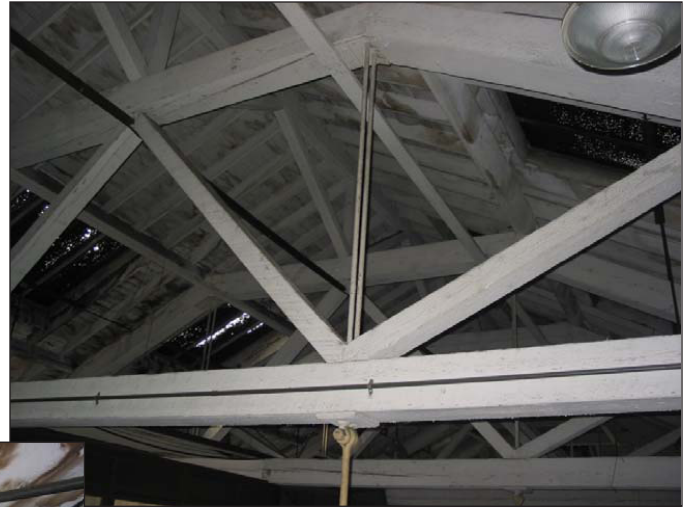
Photo 6 Below: Deteriorated Roof Sheathing (1896 Original Building)
