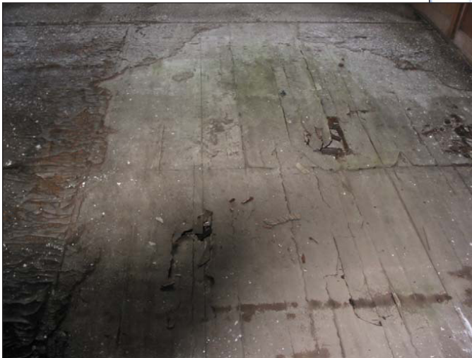
Photo 7 Below: Deteriorated 3rd Floor Finish (1896 Original Building)
