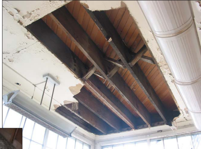
Photo 8 Above: Typical Framing at 2nd Floor (North Annex)
