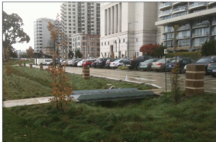
VEGETATED SWALE FOR PARKING LOT STORM WATER
