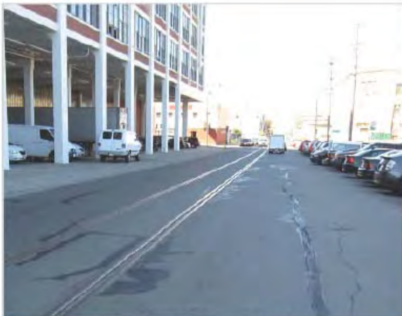
Inconsistent Parking and Sidewalk Conditions
