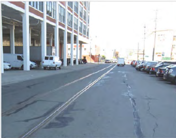
Inconsistent Parking and Sidewalk Conditions
