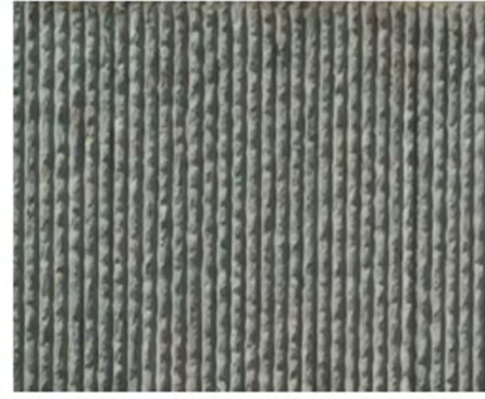
Concrete - form finished
