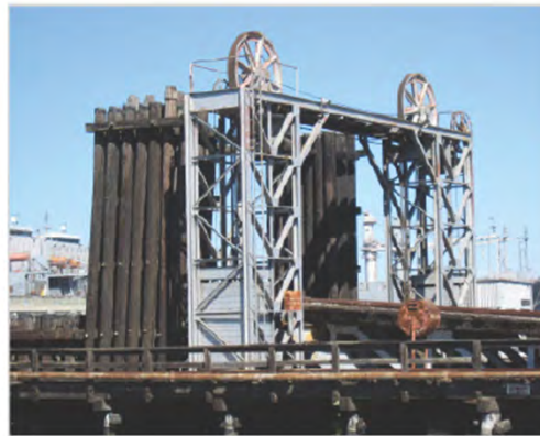
Historic Crane at Pier 70
