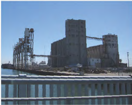
Grain Silos at Islais Creek
