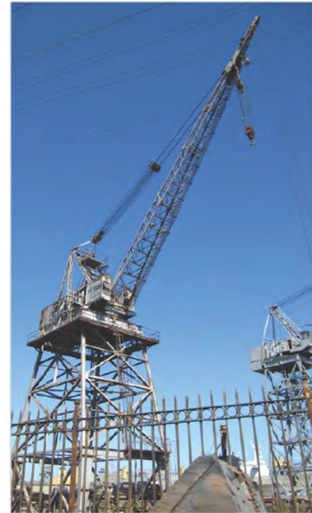
Historic Crane at Pier 70
