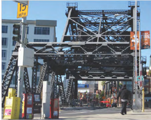
Lefty O'Doul Bridge
