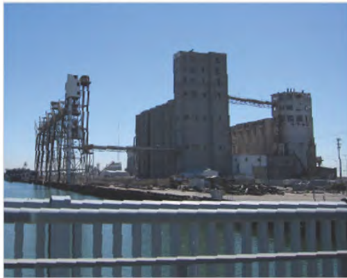
Grain Silos at Islais Creek
