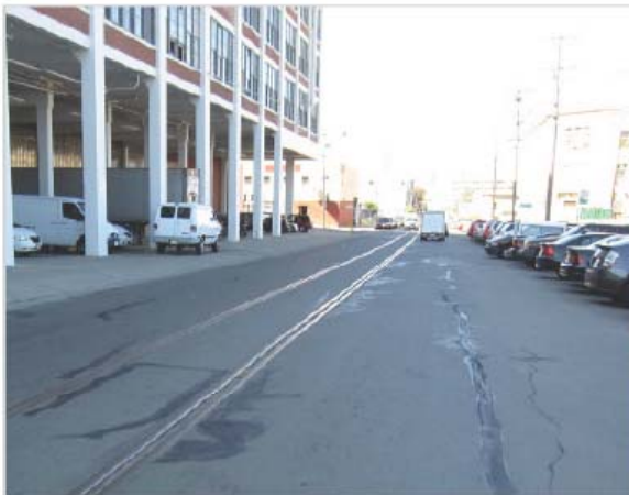
Inconsistent Parking and Sidewalk Conditions
