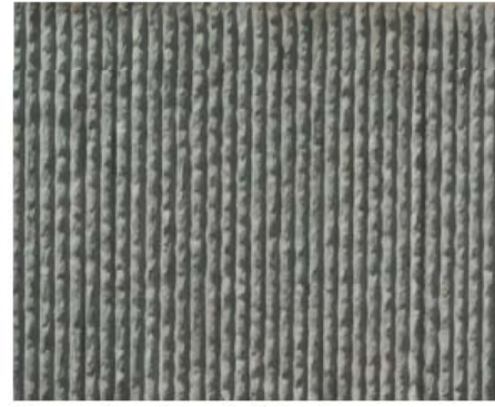
Concrete - form finished
