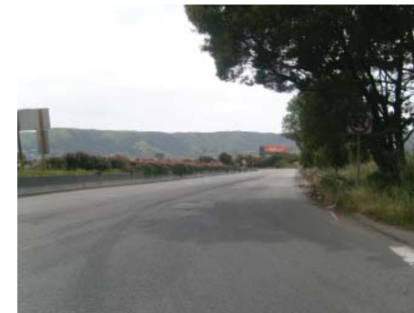
Harney at Thomas Mellon looking south
