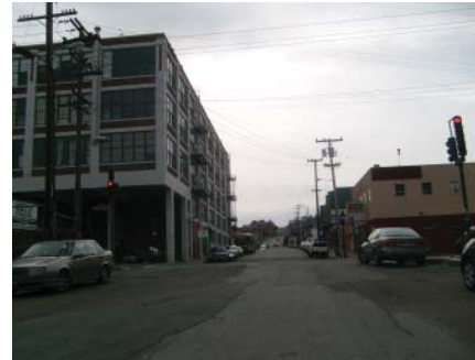
20th and Illinois looking west
