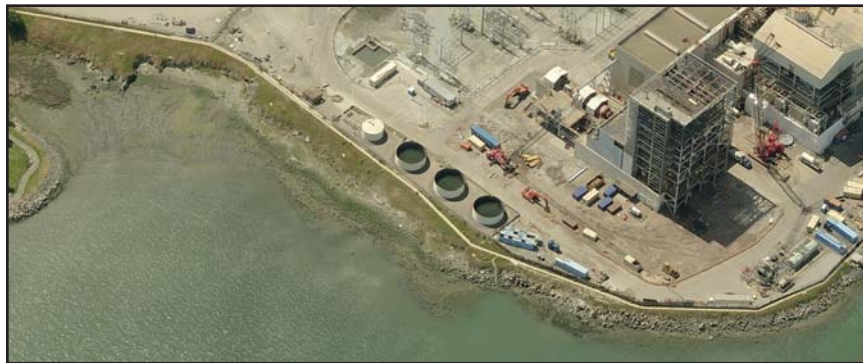
PG&E Shoreline Aerial View Facing West
