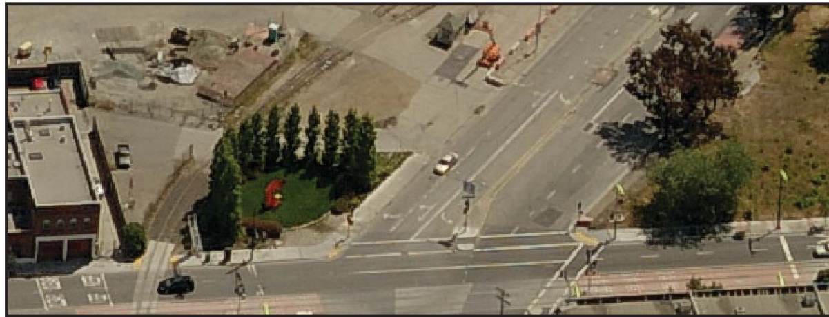
Bayview Gateway Aerial View Facing East
