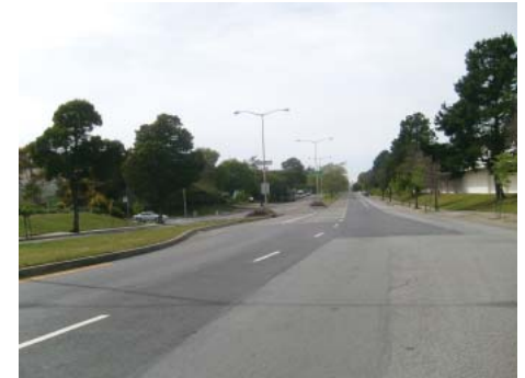
Evans at Jennings looking west
