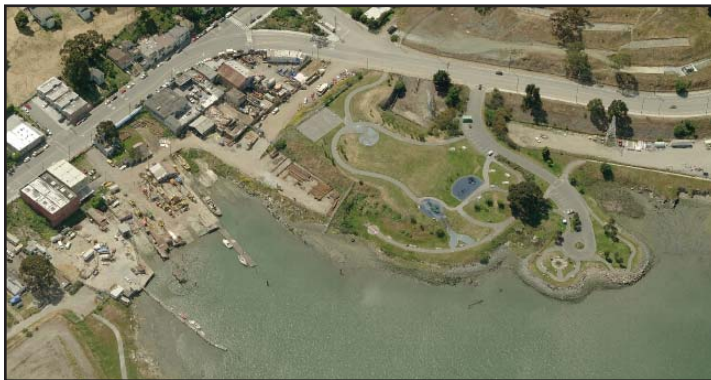
India Basin Shoreline Park Aerial View Facing West
