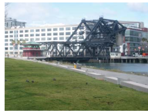
Third Street Bridge
