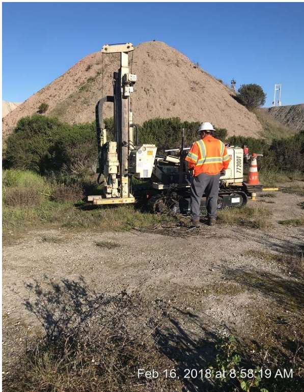
Cascade Drilling setting up over borehole AEW-7
