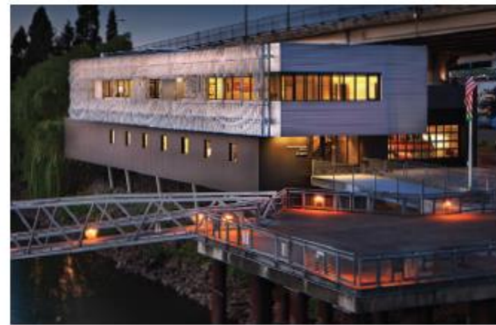
Portland Fireboat Station
