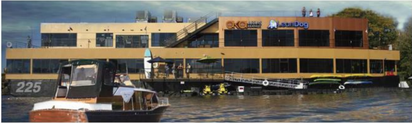
Barge 225 Floating Offices (Cleveland, OH)
