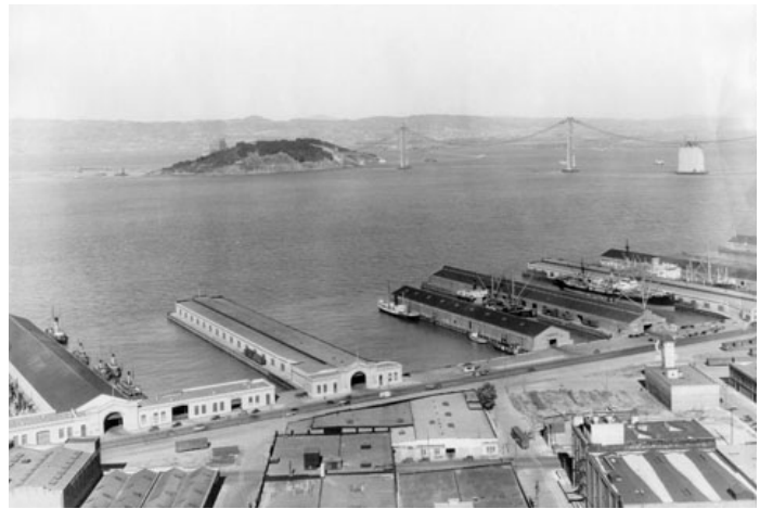
Piers 21 through 17 with the Bay Bridge under construction in the background, 1930s Source: San Francisco Historical Photograph Collection, SFPL
