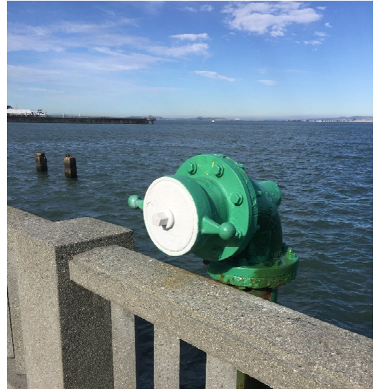
Suction connection for emergency firefighting, Rincon Park
