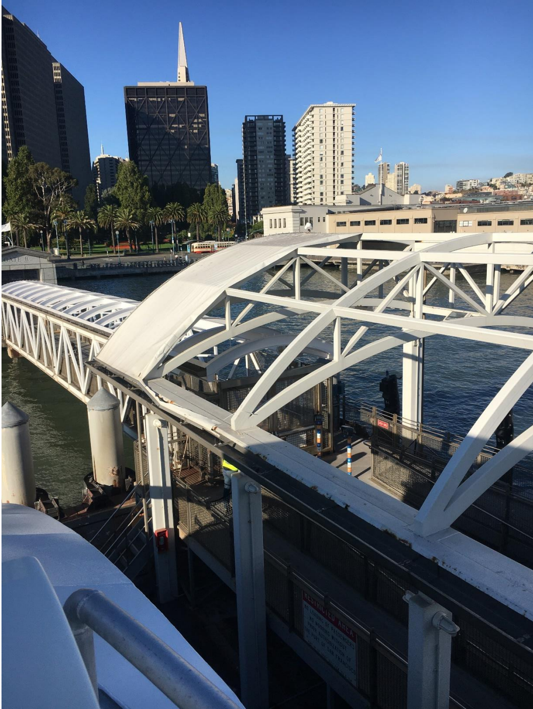
Contract No. 2820, Downtown Ferry Terminal Gate B Canopy Repair Project
