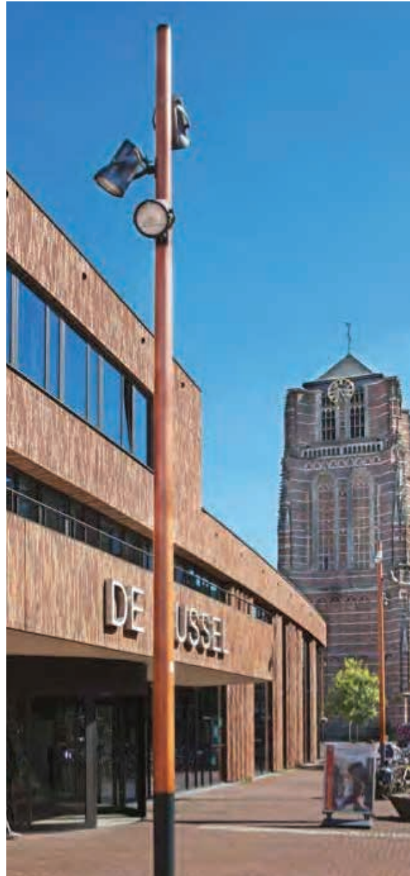
MASTS WITH MULTIPLE FIXTURE HEADS FOR MULTIPLE LIGHTING REQUIREMENTS
