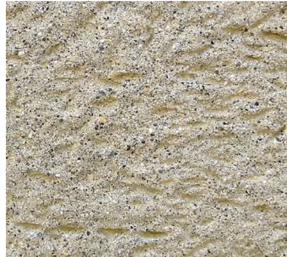
CAST IN PLACE CONCRETE WITH SURFACE TREATMENT
