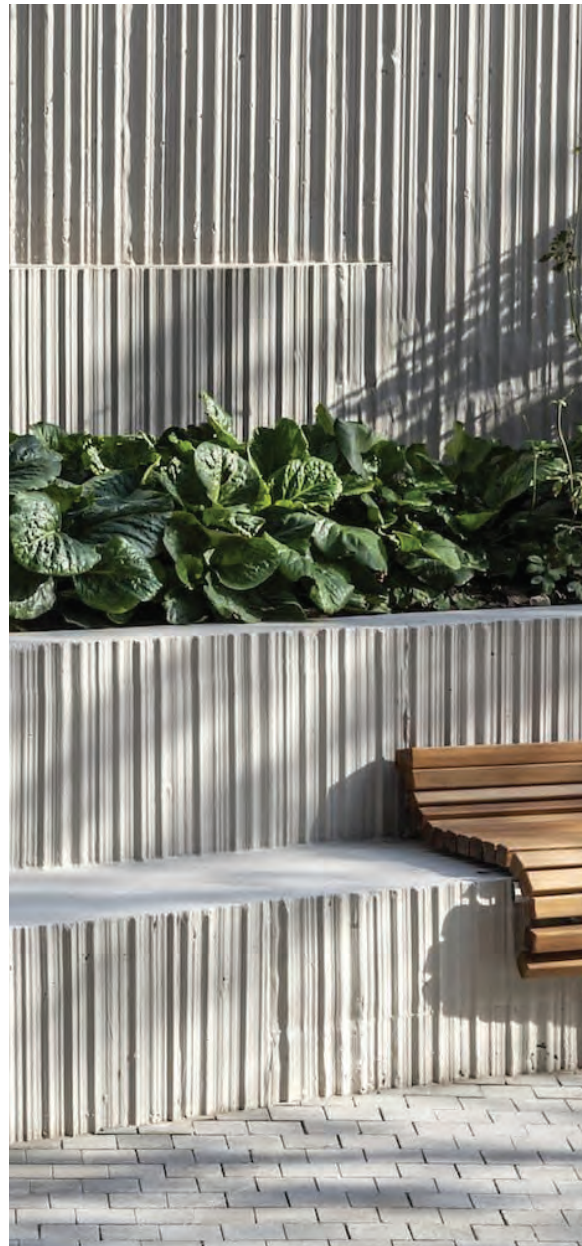
CAST IN PLACE SEAT WALLS
