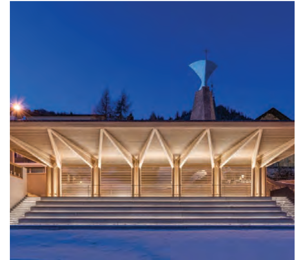
GLOW FROM STRUCTURE
