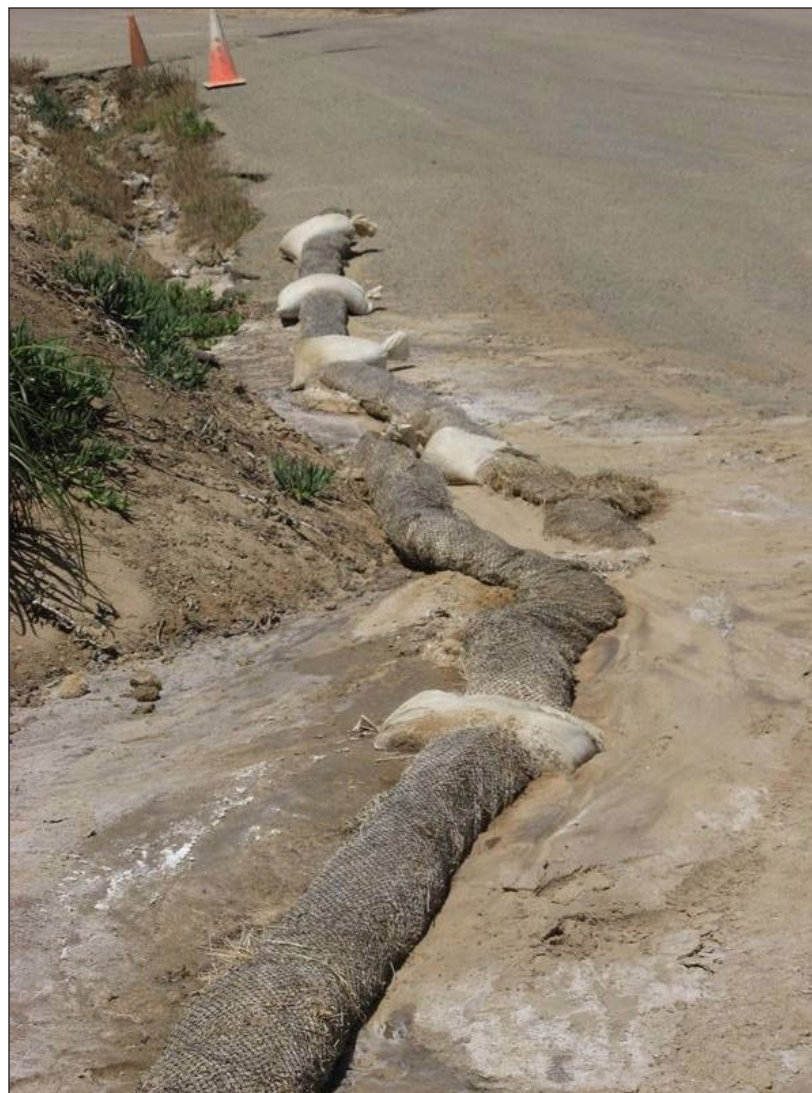
Poorly implemented and unmaintained erosion and sediment controls can lead to pollutant discharges.
