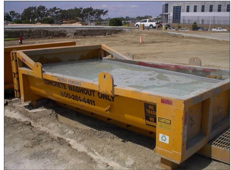
A designated concrete washout area will contain washout water and prevent it from leaving the site or entering the storm drain system.
