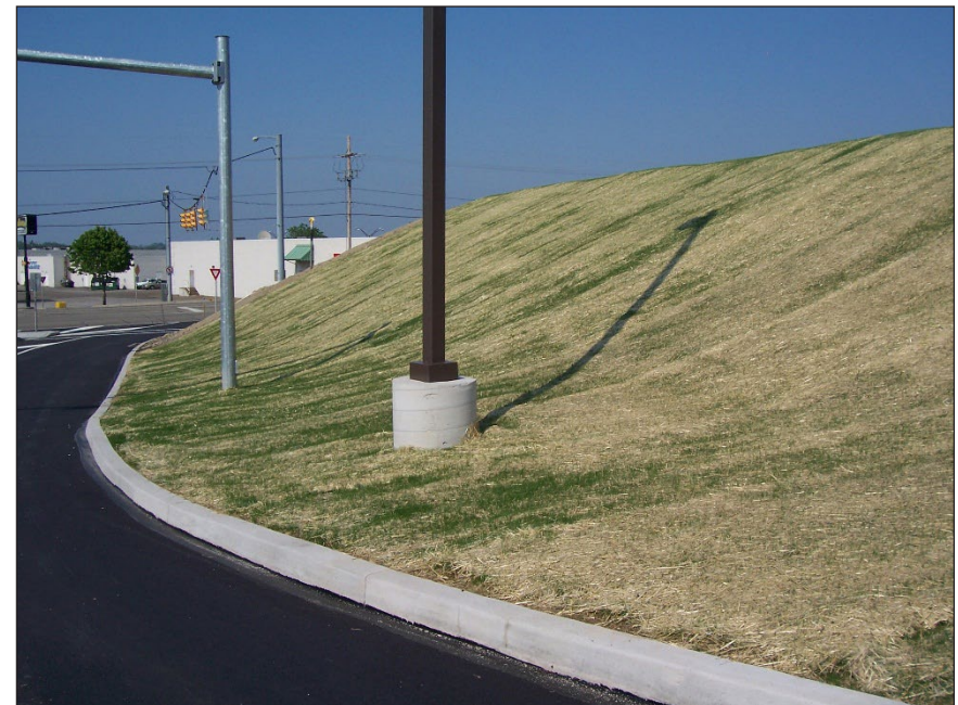
Hydroseeding protects slopes from erosion.
