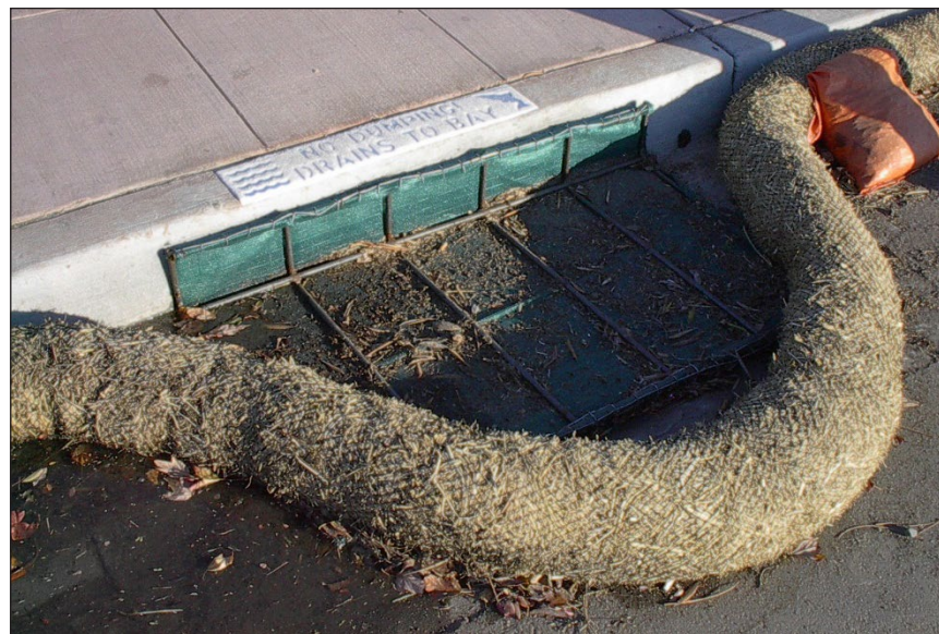
Inlets can be protected from construction wastewater using a variety of methods
