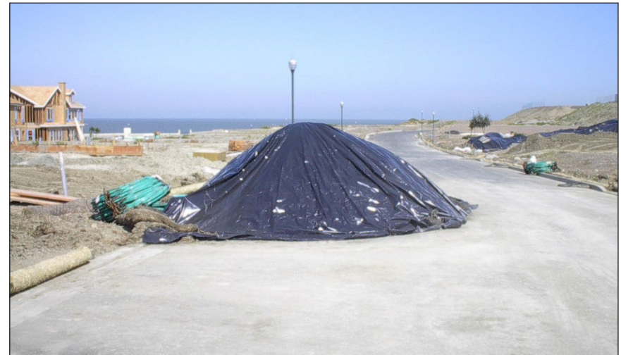
Stockpile covers should be inspected before and after rain events.
