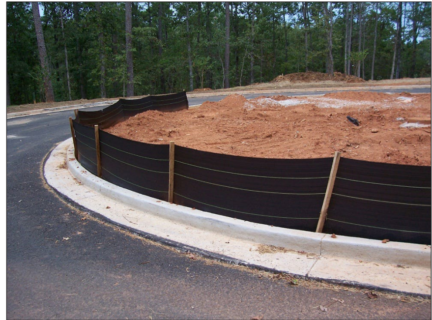
Silt fence can be used to contain sediment from disturbed areas.
