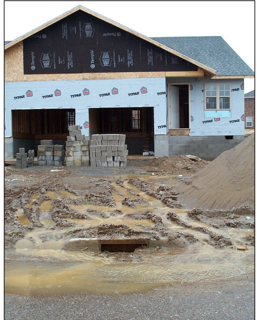
Polluted wastewater from construction sites can enter the storm drain system if erosion and sediment controls are not used properly.
