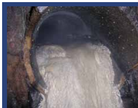
The sewer lateral, connected to a restaurant in San Francisco, is clogged by FOG.
