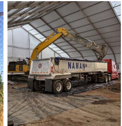
Pier 94 truckloads will be taken to nearby rail, as possible
