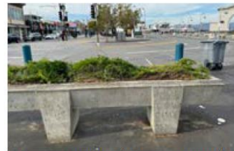
Concrete Planter (to be replanted)
