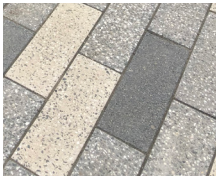
Sidewalk unit pavers (Maryland St)
