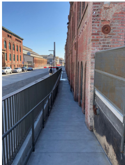
20th St. retaining wall fronting Bldg. 113
