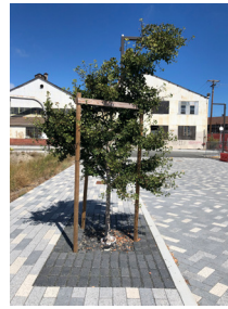
Tree well paving detail (Sitewide)
