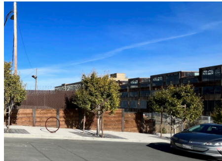
22nd retaining wall fronting Hoedown Yard
