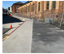
Off-street bike path paving at Bay Trail (20th St.)
