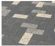
In-Street Unit Pavers (Maryland St)
