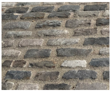
Parking Lane & Crosswalk Cobbles (20th St)
