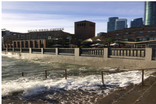
Figure 15: King Tides flooding at Pier 14
