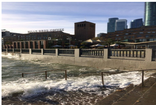
Figure 15: King Tides flooding at Pier 14
