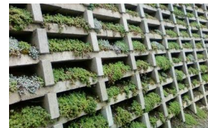
Vegetated Crib Walls
