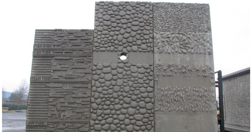
Seattle seawall's textured face panels before installation - Seattle, WA. ©Seattle DOT via Flickr.com
