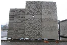
Ecological Concrete Structure
