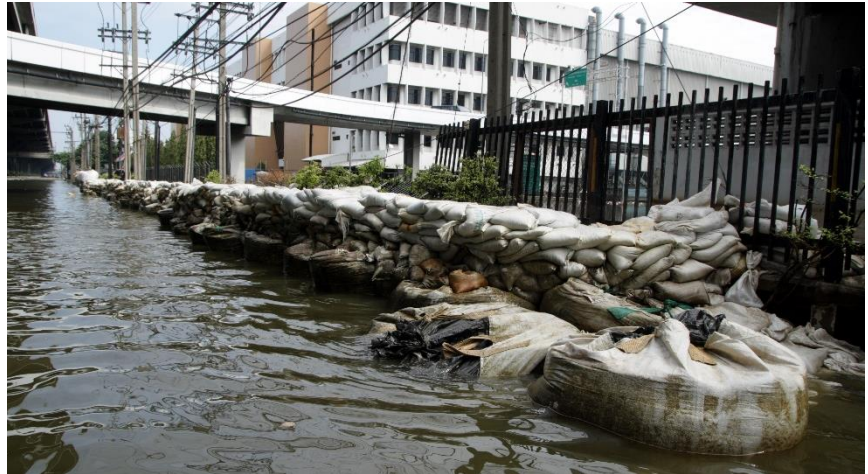
Sand bags line on street protected from floodwaters - Bangkok, Thailand ©Shinji Makoto/Alamy Stock Photo
