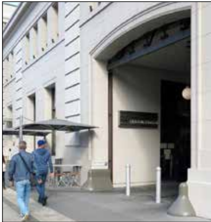
Fig. 25. Sign within Circulation Opening.
