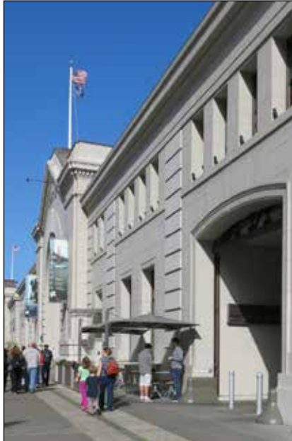
Fig. 12. Pier 3 Bulkhead Building.
