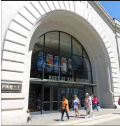
Fig. 14. Pier 1 Central Arch.
