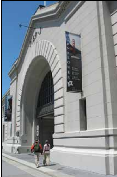
Fig. 18. Banner Signs on Pier 3.
