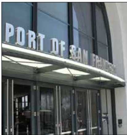
Fig. 15. Pier 1 Canopy and Signage.
