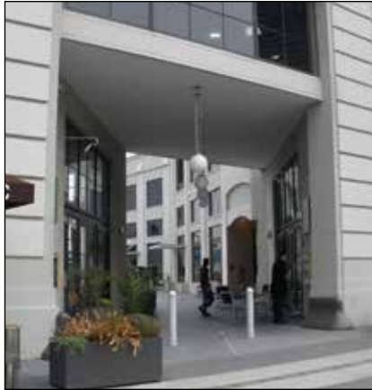
Fig. 24. Circulation Opening at Pier 3.
