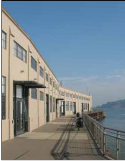
Fig. 33. Cargo Openings with Canopies on Pier 1 Shed.
