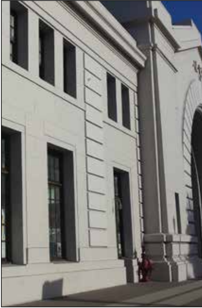
Fig. 31. Pier 31 ground-level Minor Windows.
