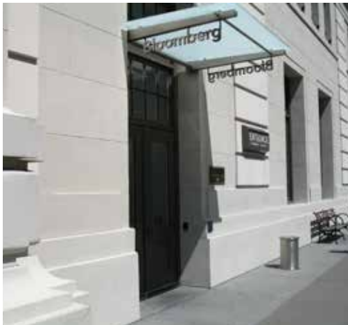
Signage and entry canopy.
