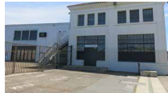
North edge of Pier 38 bulkhead building
