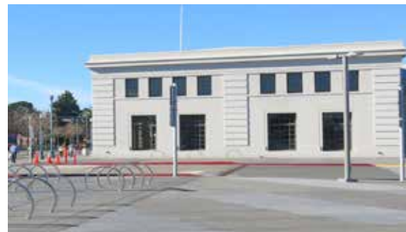
South edge of Pier 29 bulkhead building
