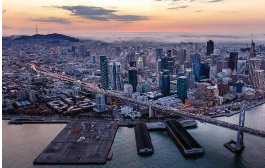
Piers 30-32 and SWL 330 on the Port of San Francisco waterfront
