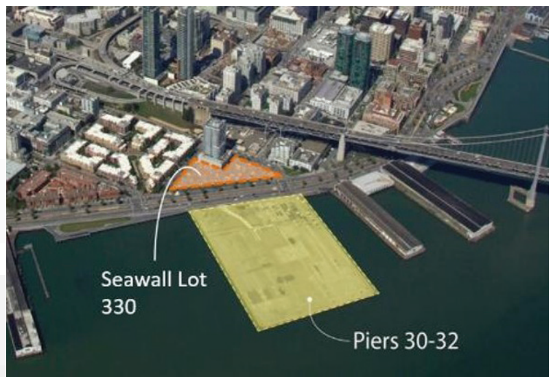
Aerial view of Piers 30-32 and SWL 330
