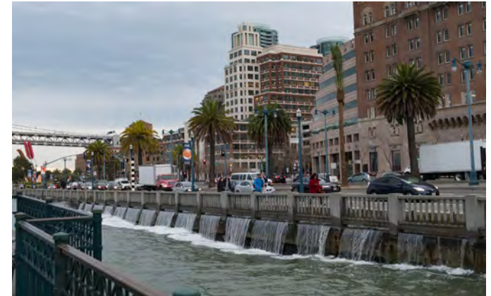
Flooding along the Embarcadero Seawall
