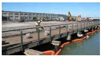
Floating boom is deployed around construction work to capture debris.
