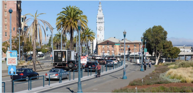
Two-way Class IV bikeway installed with quick-build treatments in 2020/2022
