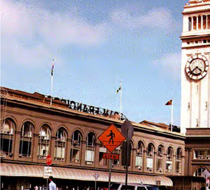
1996, EXTERIOR TREATMENT OF ARCADE
