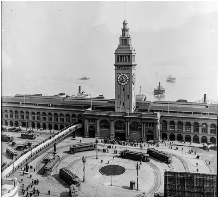
1930, PEDESTRIAN BRIDGE INTRODUCED
