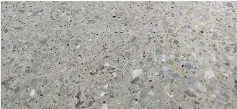
EXISTING CONCRETE GROUND & SEALED
