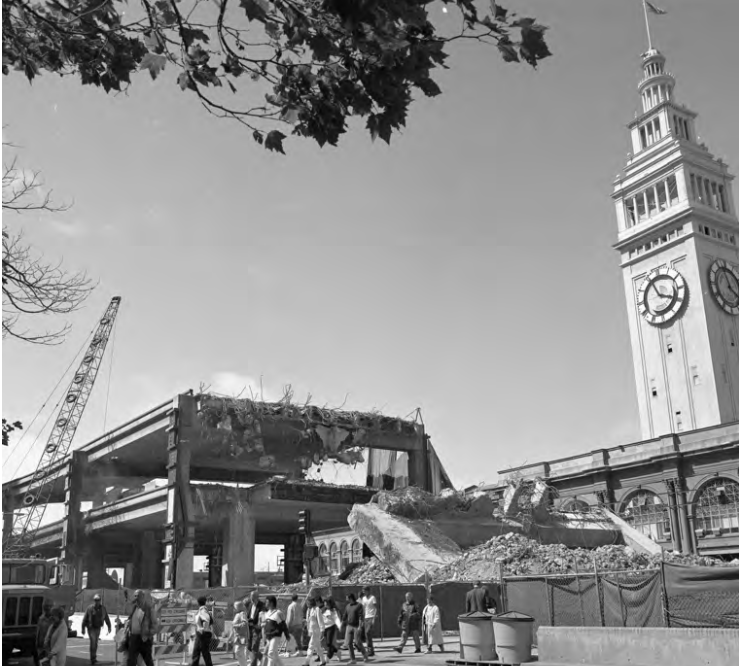
1991, DEMOLITION OF EMBARCADERO FREEWAY
