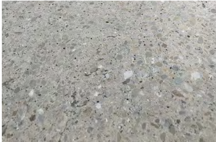
EXISTING CONCRETE GROUND & SEALED
