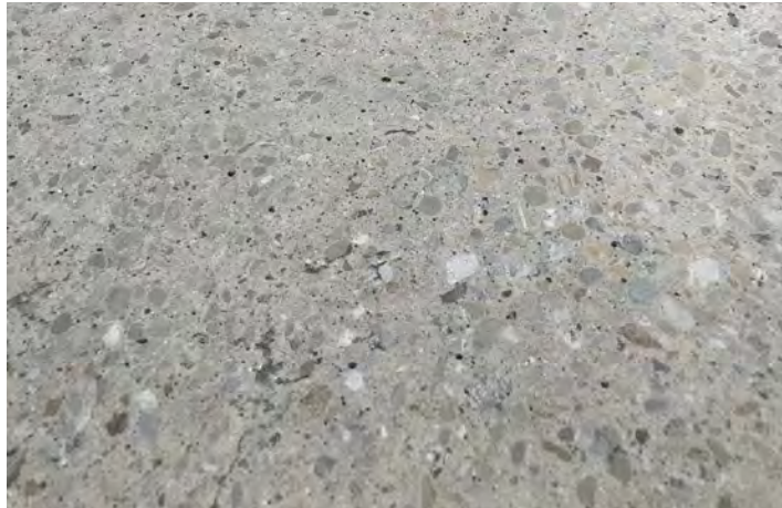
EXISTING CONCRETE GROUND & SEALED
