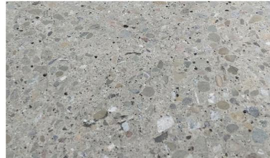
ECOGRIND TREATMENT AT EXISTING PAVING BANDS
