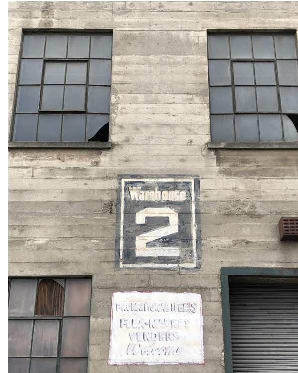
Detail: Board-Form Concrete & Painted Signage
