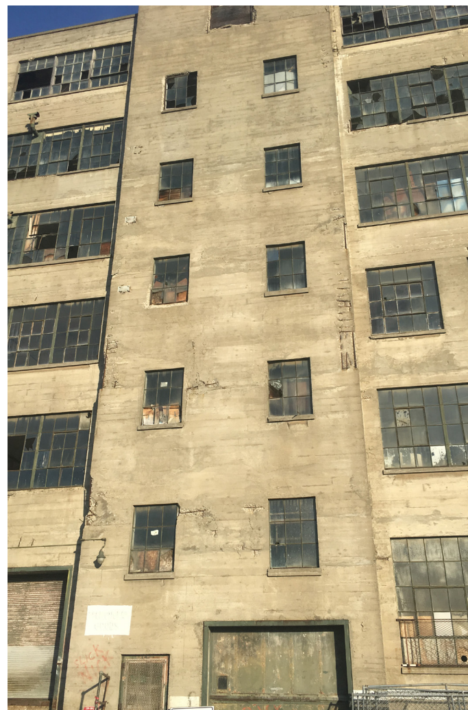
View of Stair/Elevator Tower Condition
