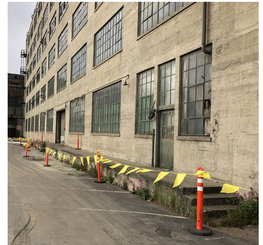
East Elevation with Loading Dock
