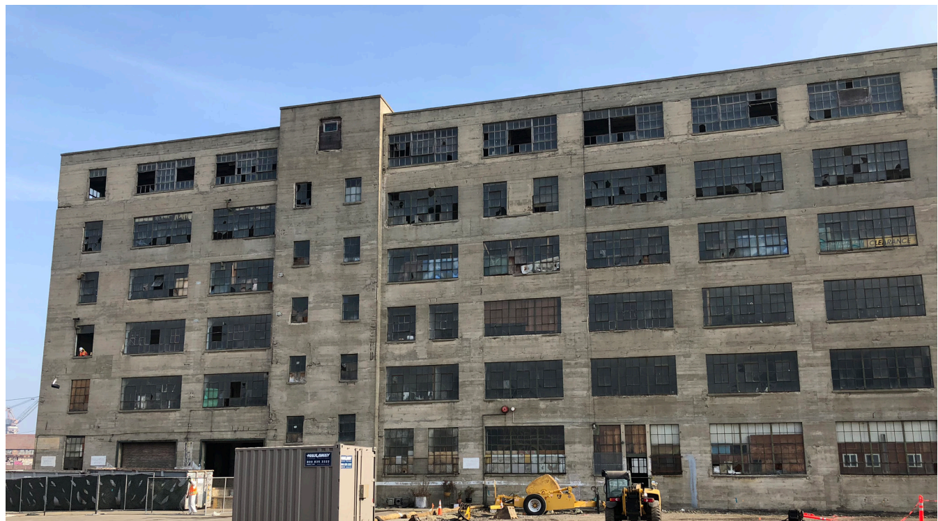
West Elevation with Stair/Elevator Tower
