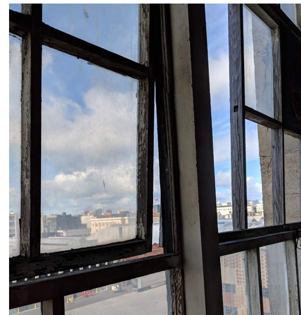
Detail: Level 6 Wood Sash Window
