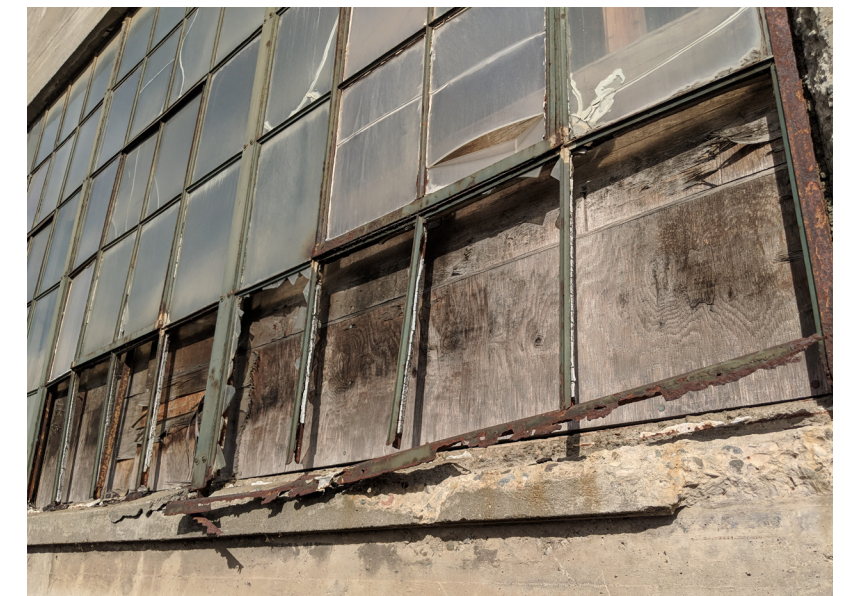
Detail: Example of Window Condition
