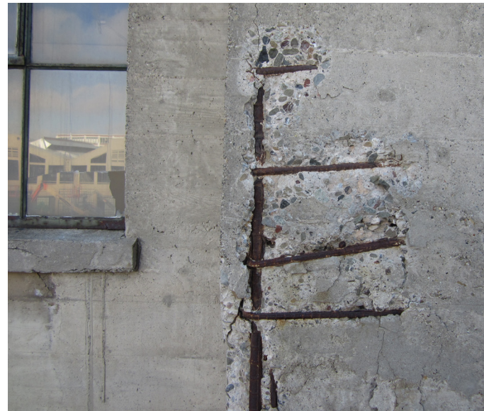
Detail: Example of Facade Condition
