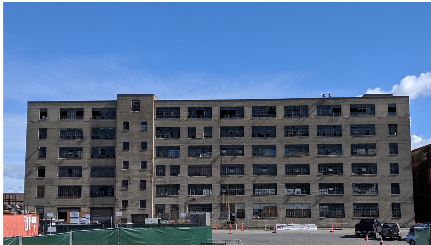
West Elevation with Stair/Elevator Tower
