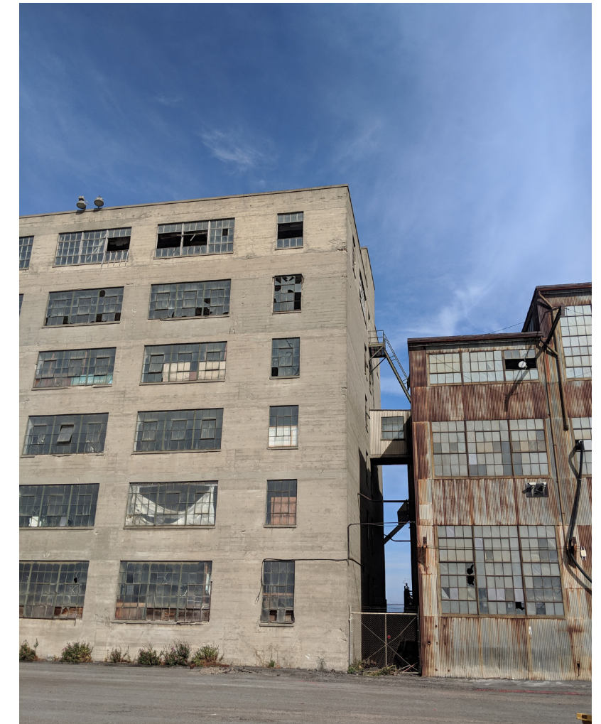
View of Connection to Building 12
