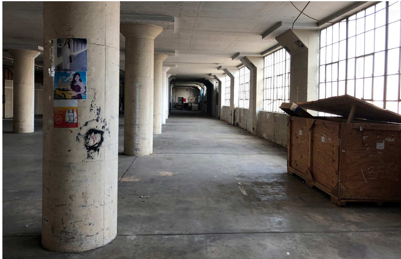
Interior View of Columns
