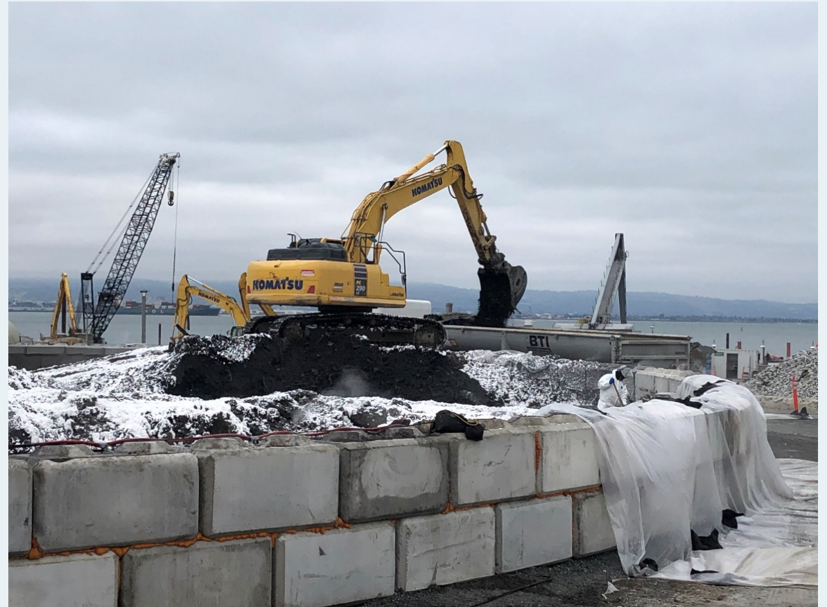
SF Potrero MGP Remediation Project - Material Handling Operations
