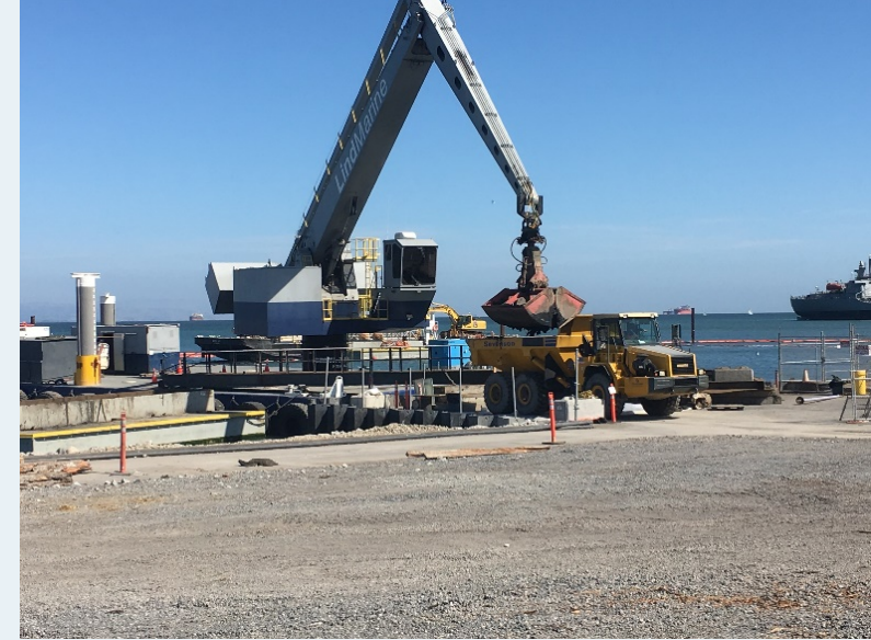
San Francisco Potrero MGP remediation project – Sediment Offloading Operations
