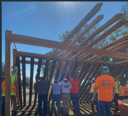
Volunteering with Rebuilding Together
