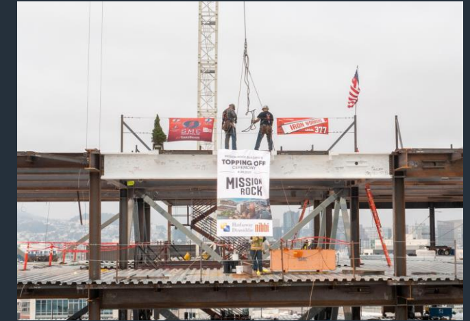
Visa Building Topping Off Ceremony
