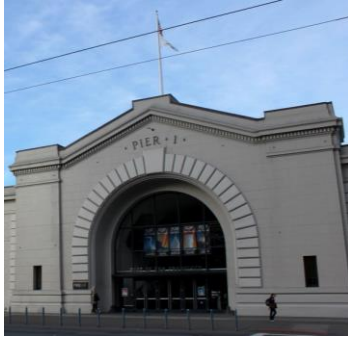
Bulkhead Wharf Retrofits
