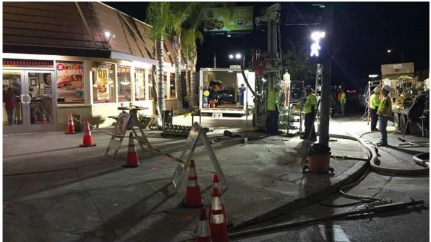
Installation at night © Fugro and SGH
