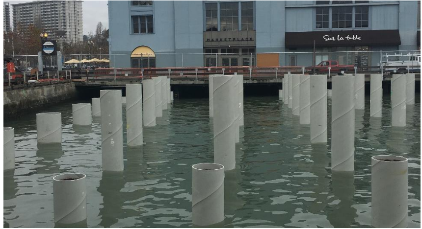
Example of piles installed to support new wharf structure ©SGH
