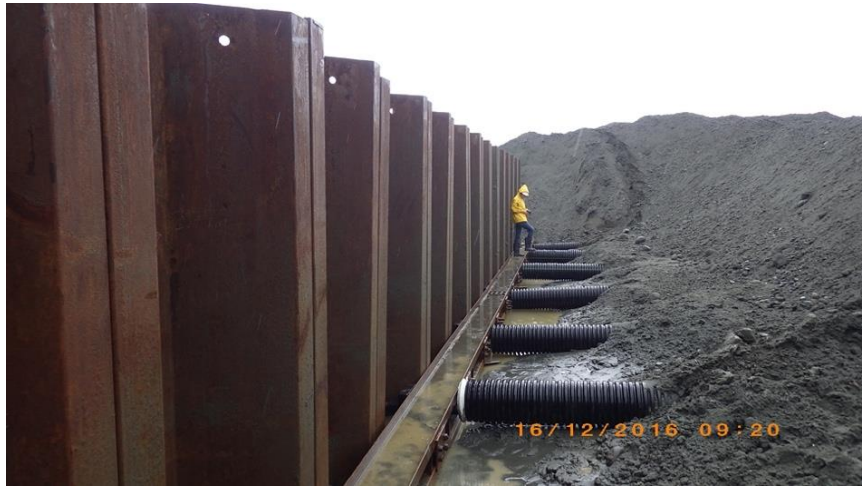
Example of sheet pile and filling operations @Jacobs
