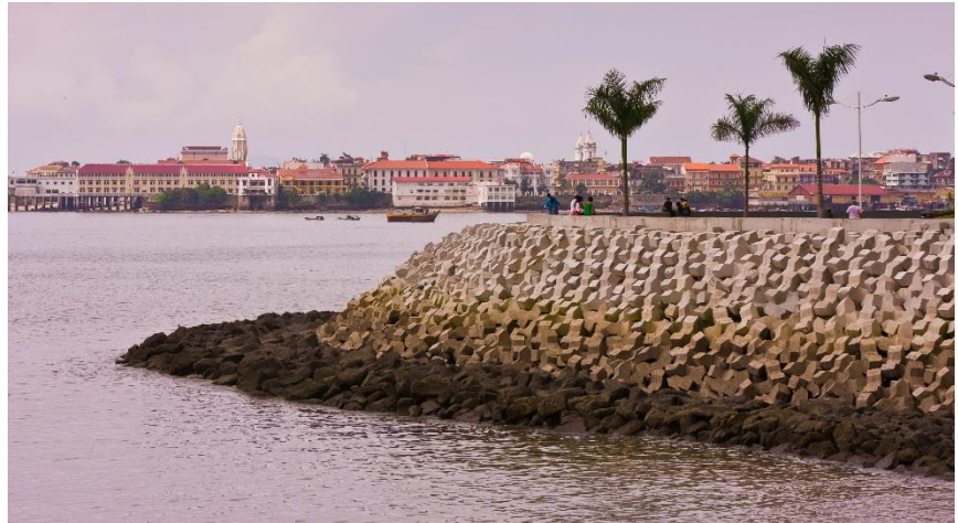
Seawall of riprap on Panama Bay - Panama City, Panama ©Rob Crandall/Alamy Stock Photo
