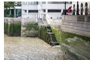
New Seawall Bayward
